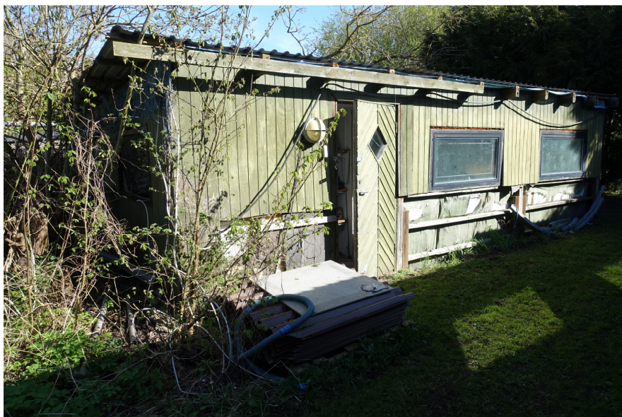
Billede 10 Udhus (bygning F).
