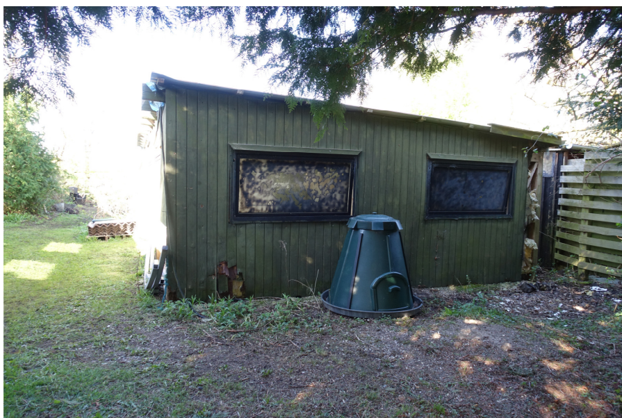
Billede 11 Udhus (bygning F).
